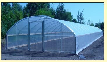
20 x 96 Low Profile Quonset 4' Sides 5' On Center 20 - Bows 1 5/8" 14 ga. 40 - 6' Legs 1 7/8" 15 ga. 1 - 96' Purlin 1 3/8" 16 ga. 4 - 21' End Braces 1 3/8" 16 ga. Hardware to assemble
